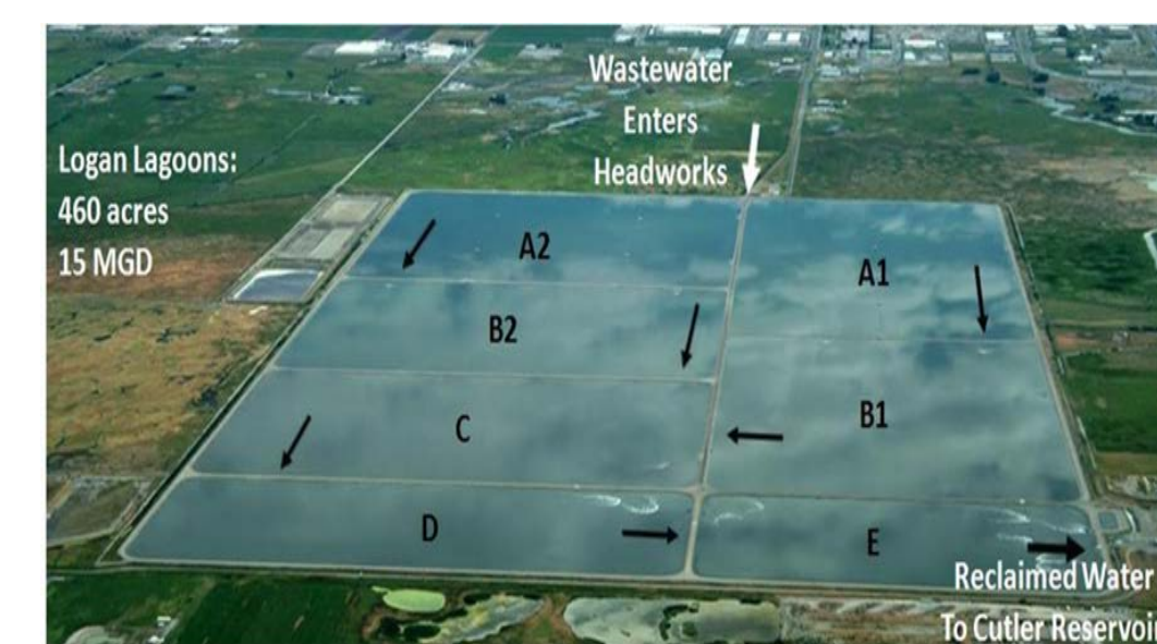
Figure 1: Logan Utah Wastewater Treatment Plant
