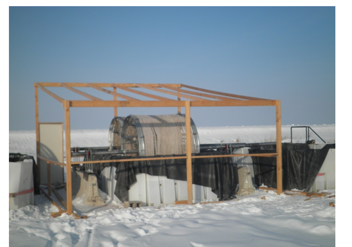
Figure 13: Greenhouse during construction
